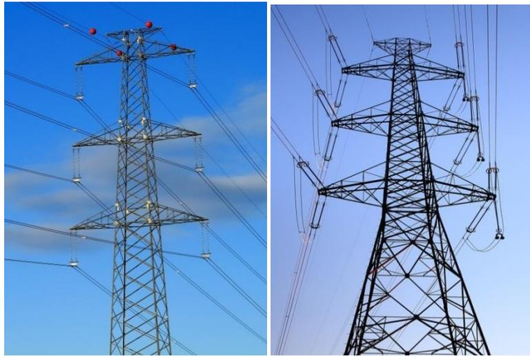
Figure 5-3: Line carrier pylons and anchor masts for 400 kV aerial conductor
