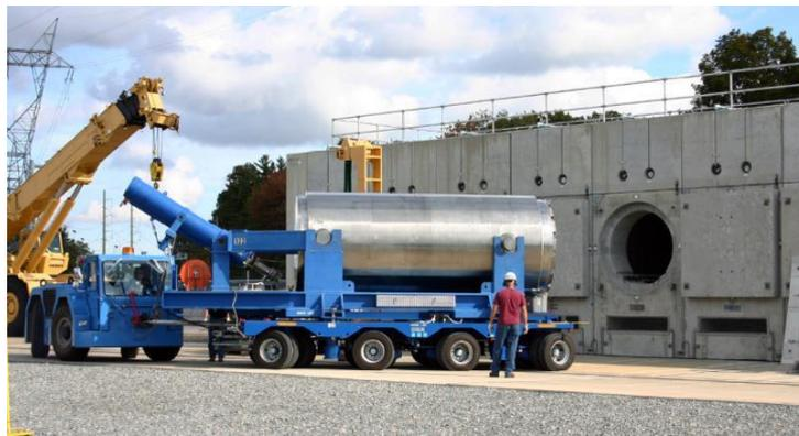
Figure 19.4.2-6.: Filling the cask for dry storage, lying layout. [19-37], [19-38]
